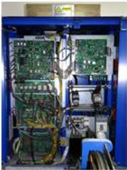
Inverter for elevator
